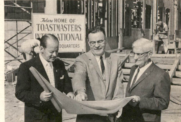
Executive Director Maurice Forley, President Herman Hoche and Dr. Smedley inspected the progress of the World Headquarters building in November, 1961.
