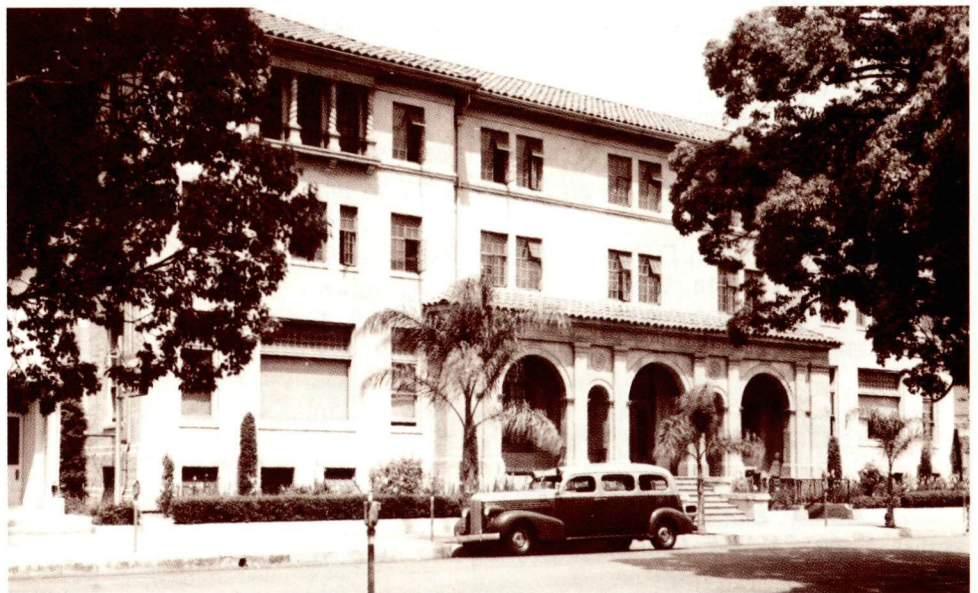
Toastmasters today and yesterday—Today's stately World Headquarters building in Santa Ana, California (left), provides a modern contrast to the stateliness of Toastmasters' first home, the Santa Ana YMCA (above).
